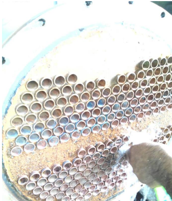
Condenser tubes during flushing after chemical cleaning
