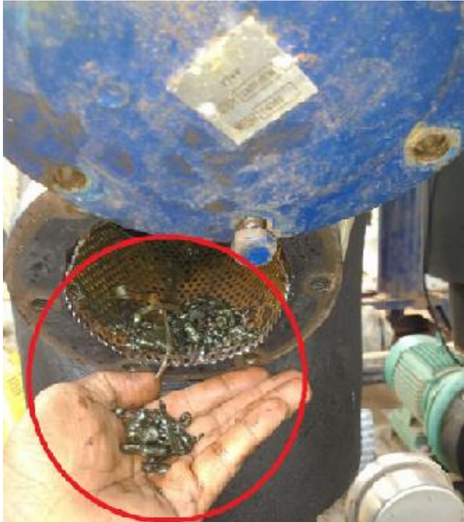
Welding Flux, Iron Fins and Pre – fabrication debris during Chemical flushing
